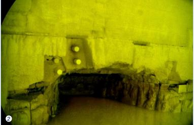
Figure 3 shows the situation after the hot face welding has been completed. The missing material has been replaced and the new material is completely bonded with the remaining existing refractory.
