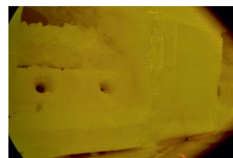
Situation during ceramic welding 燃烧器墙焊中
