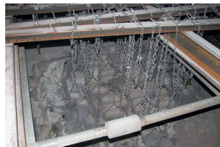
After welding from outside 焊接外部后
