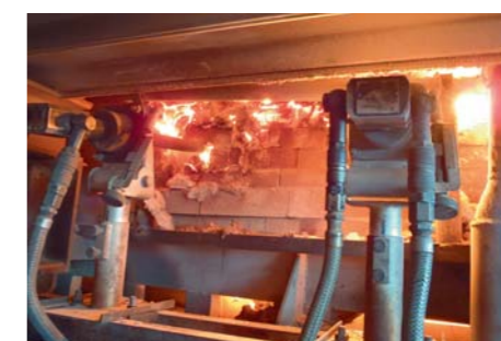
Situation before from outside 燃烧器墙焊前
