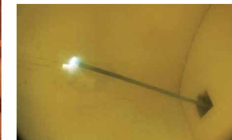
Welding of the crown 炉顶焊接
