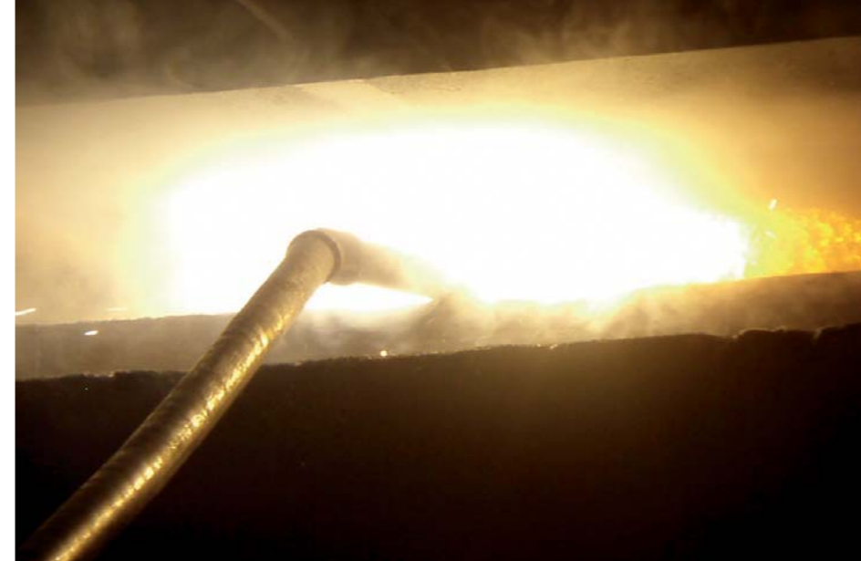
During welding process 焊接作業中
