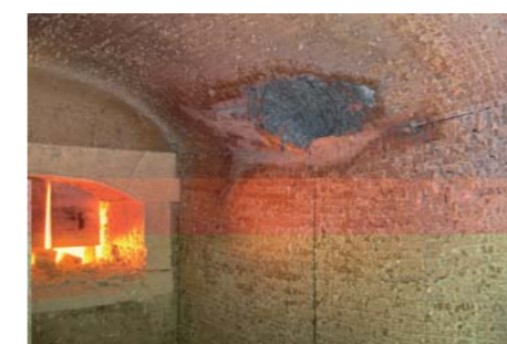
Regenerator crown after cooling down 冷却后的蓄热室顶
