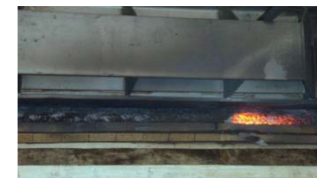
Cooling down of welding material 焊材冷卻
