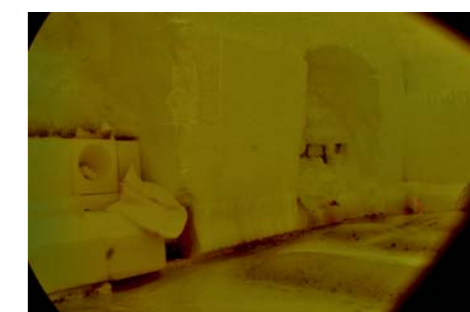
Situation after exchange tuckstones and burner blocks 更换胸墙底砖和燃烧器砖后
