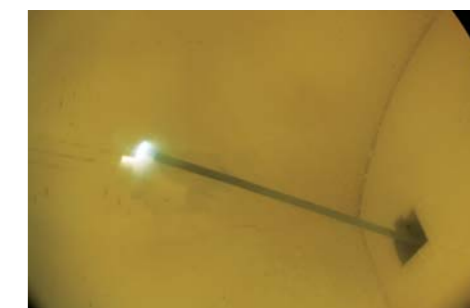
Regenerator crown during welding 蓄热室顶焊接中
