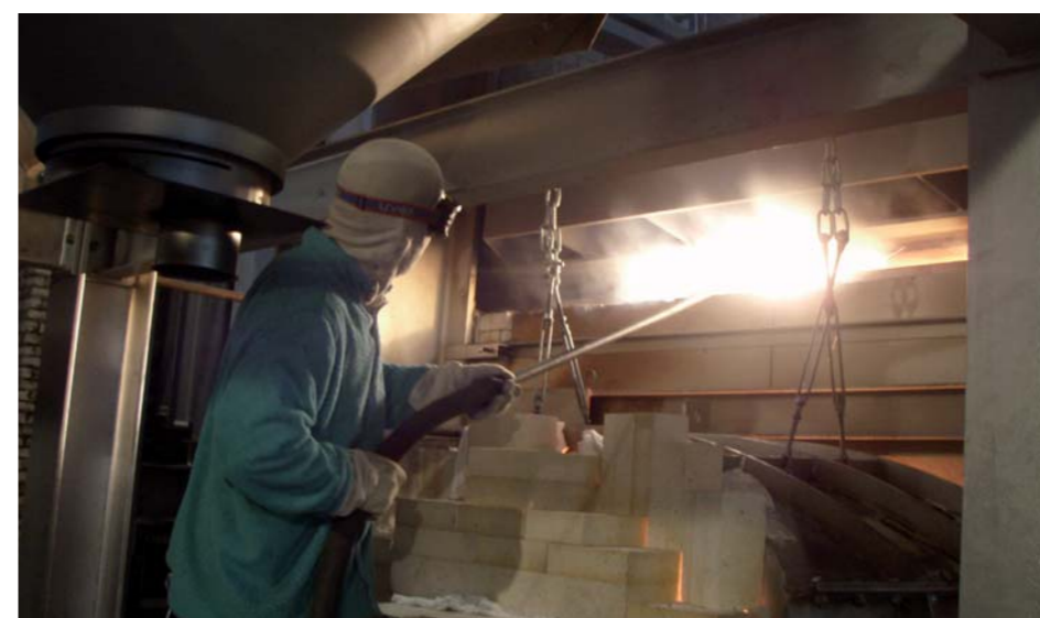
Skew back joint before welding 焊接前拱座膨脹縫
