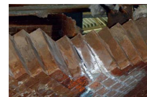
Joints after cooling down 冷却后的砖连结
